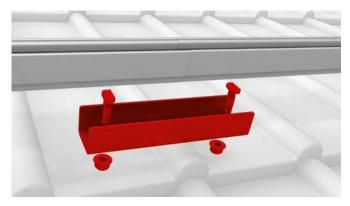
Ensure correct position of T-bolt. After inserting into the lower chamber of the rail, the T-bolt is turned 90 degrees counterclockwise. Lock the projected K2 module carrier rail Solid on the adapter plate with an M10 T-bolt and tighten. Tightening torque: 32 Nm
